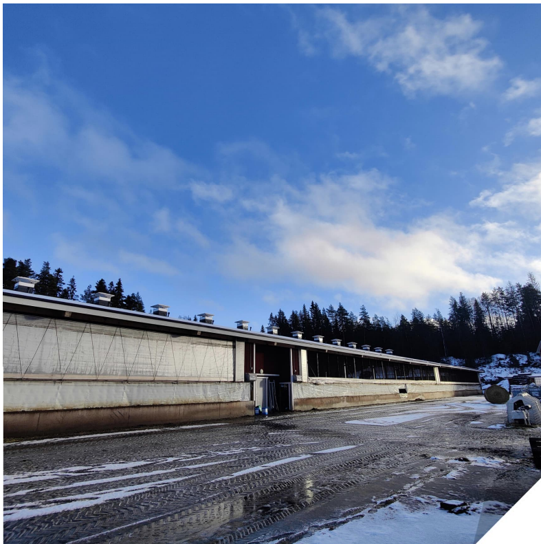
Figure 3. Side walls of the Arvela dairy barn. Curtain walls are completely open in the for the main area, but closed for the area where pregnant cows are housed. Ridge chimneys are also visible.
